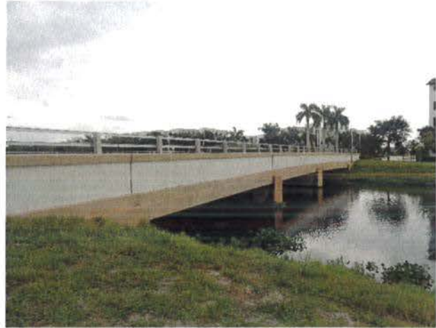
South Bound Renaissance Commons Blvd Bridge
