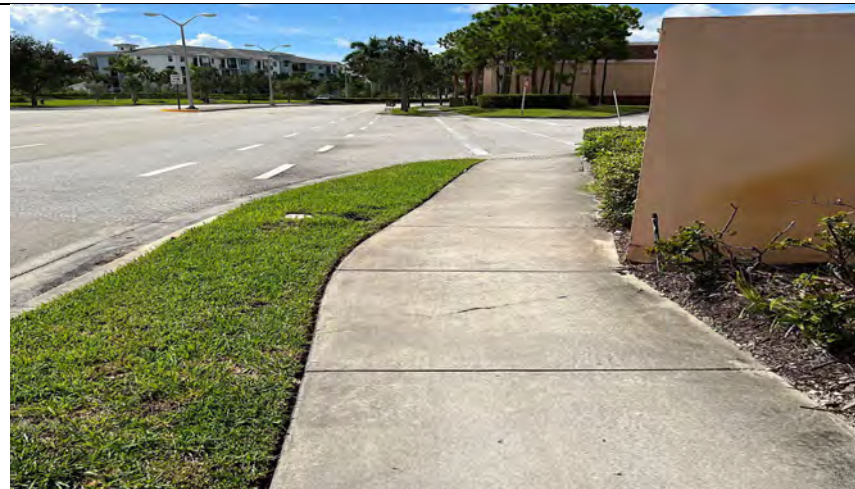
Photo 9: Broke sidewalk behind Michaels
