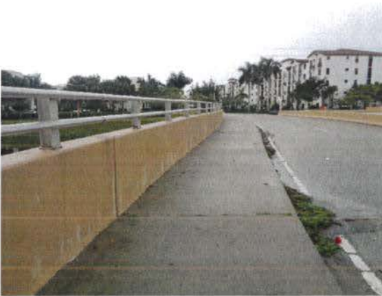
42-inch barrier wall and sidewalk on east side of bridge
