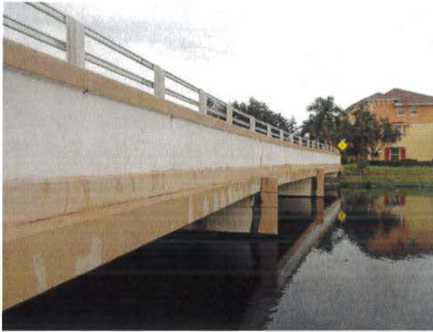
North Bound Renaissance Commons Blvd Bridge
