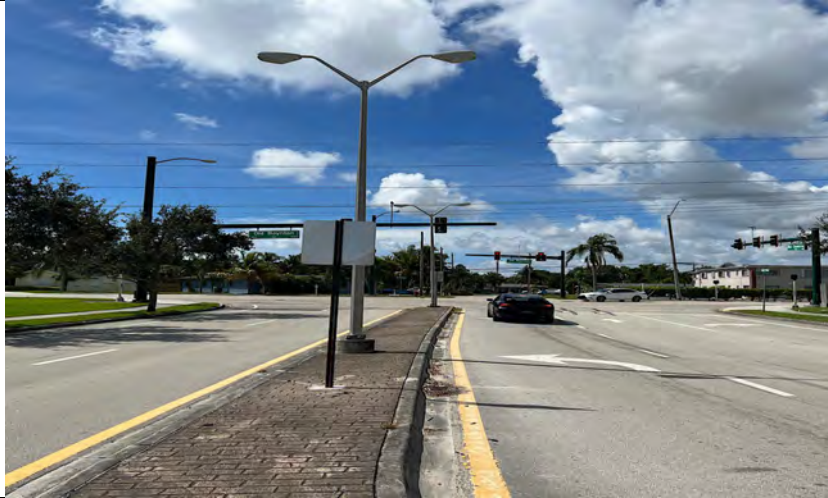
Photo 22: Left turn only sign on backwards
