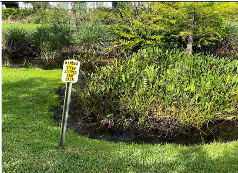
Photo 5: Steep slope sign has faded letters-outfall needs excavation
