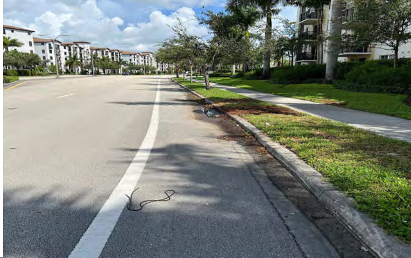
Photo 19: dirt in gutter
