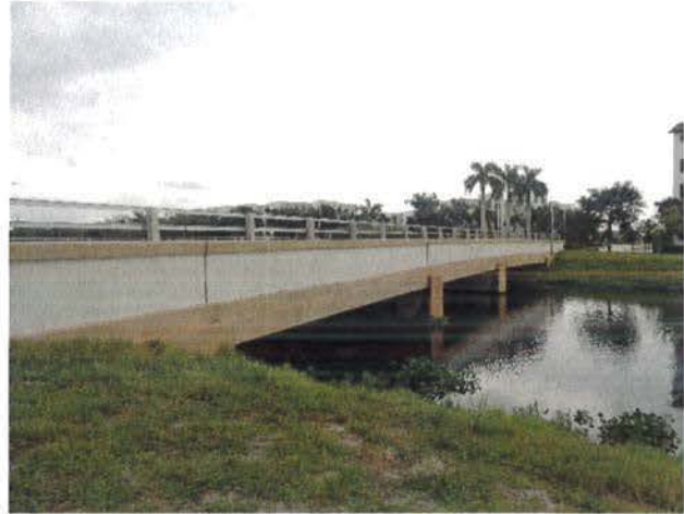
South Bound Renaissance Commons Blvd Bridge
