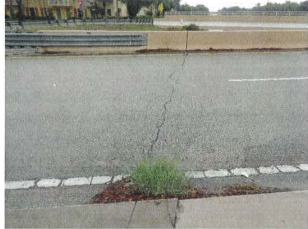
Vegetation growth adjacent to sidewalk
