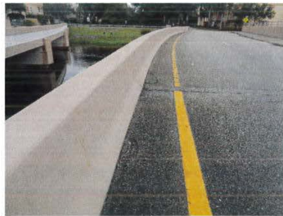
32-inch barrier wall on west side of bridge
