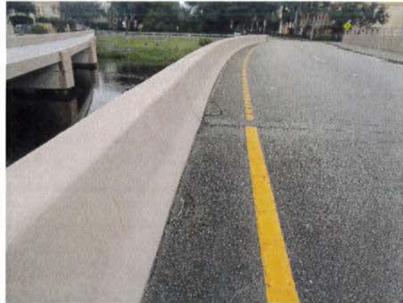
32-inch barrier wall on east side of bridge
