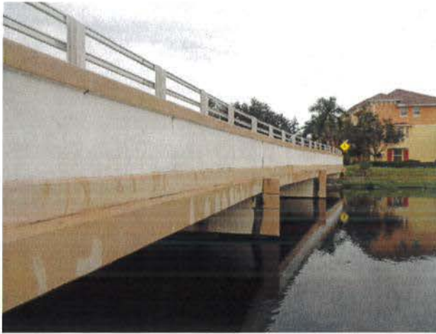
North Bound Renaissance Commons Blvd Bridge
