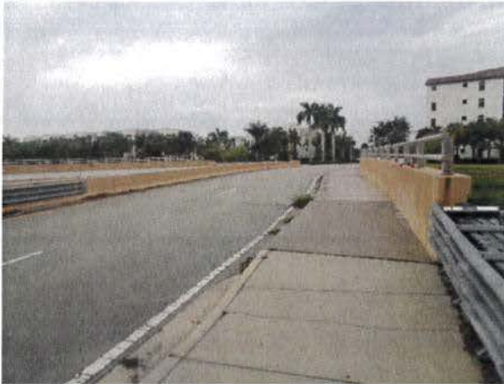
42-inch barrier wall and sidewalk on west side of bridge
