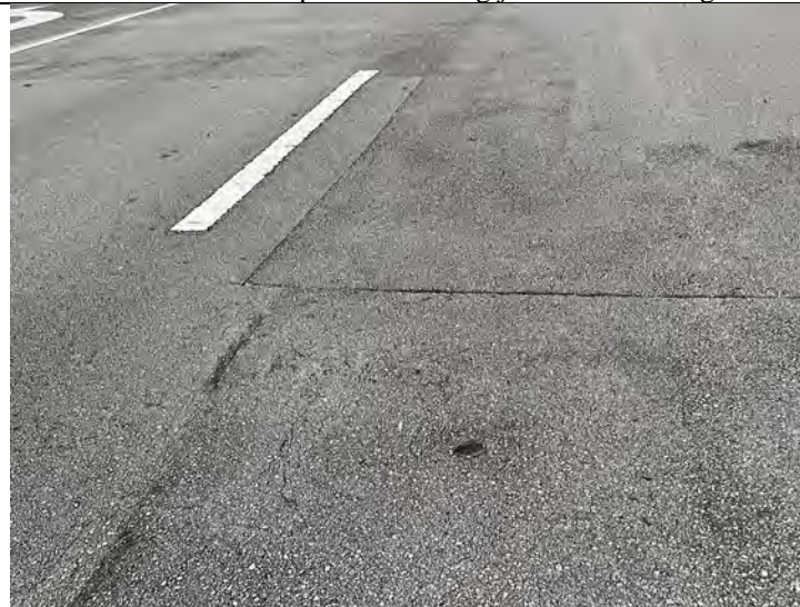
Photo 38: RCBS- small holes forming just south of bridge
