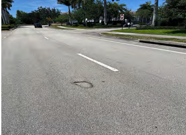
Photo 37: RCBN-pothole forming just south of bridge
