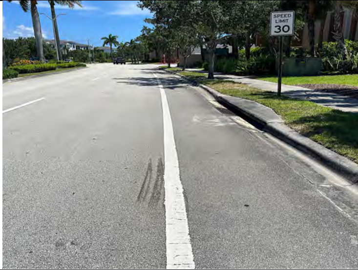
Photo 28: Gouges in asphalt RCBS
