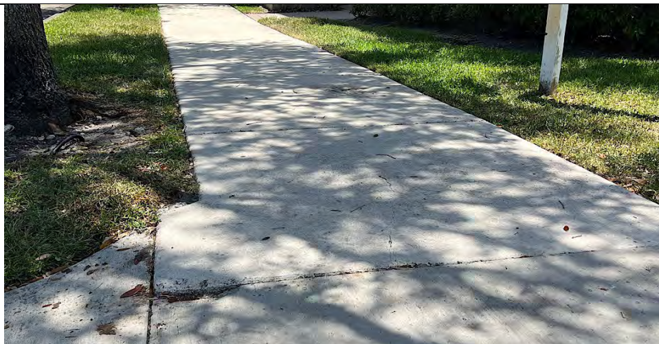
Photo 21: Trip Hazard-broken Walk south of bridge RCBS
