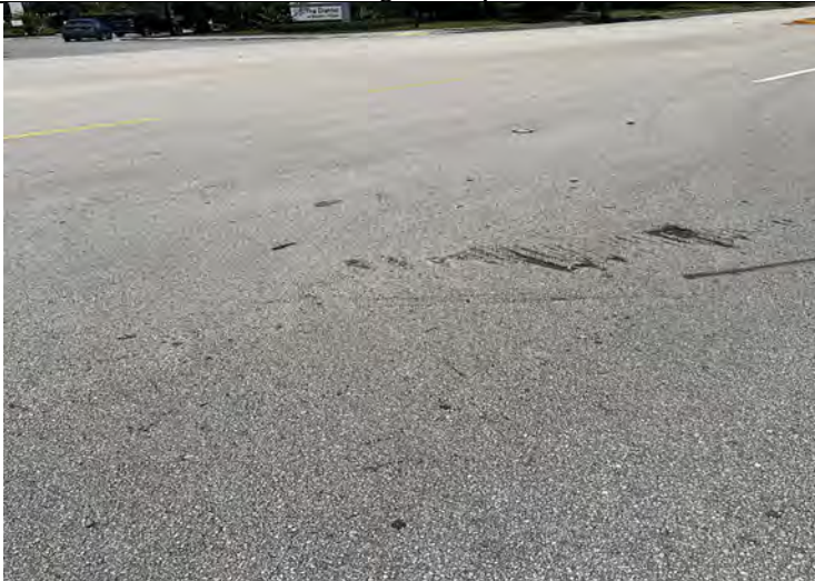
Photo 29: Gouges in road RCBS
