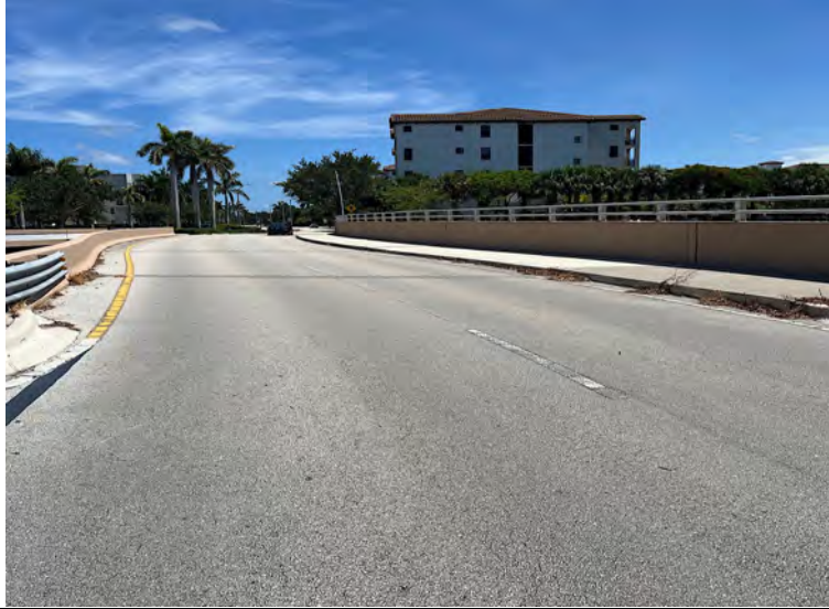
Photo 40-RCBS-dirt and weeds on bridge
