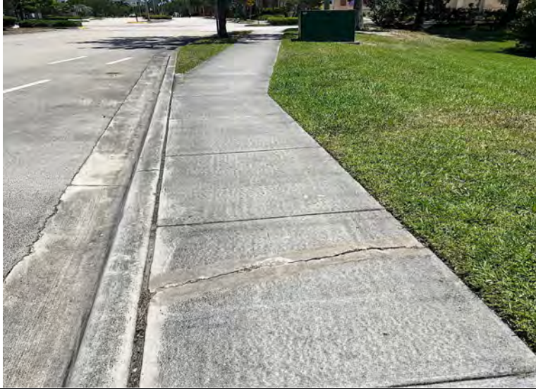
Photo 25: Broke walk in bus drop-off RCBS
