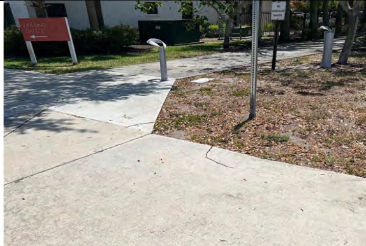
Photo 20: Broke Sidewalk-Trip Hazard south of bridge RCBS
