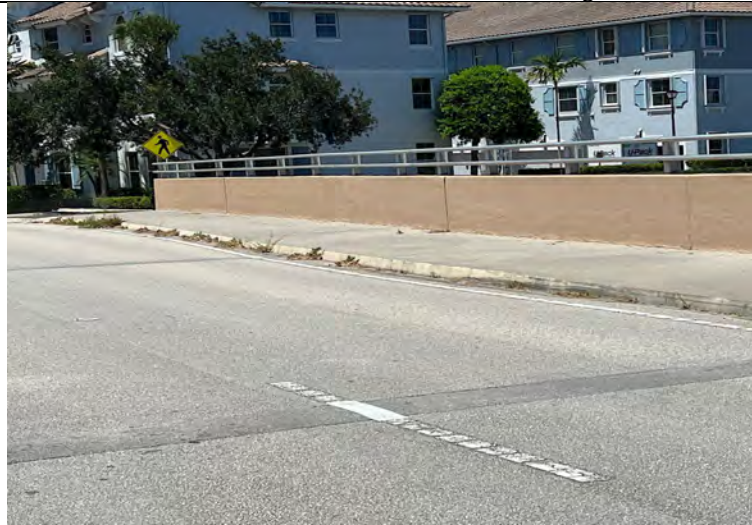
Photo 41-RCBN-dirt and weeds on bridge
